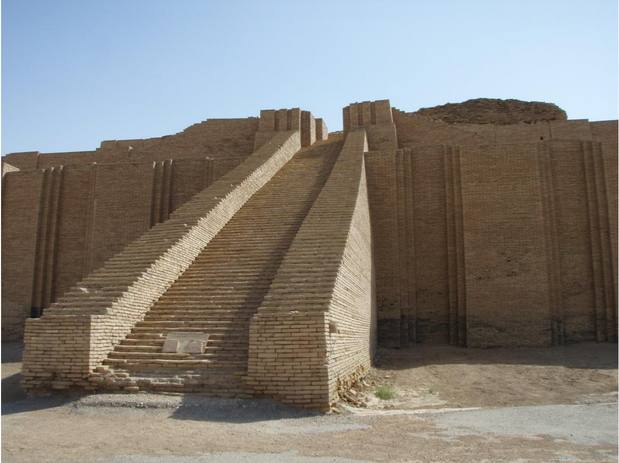
Ziggurat of Ur (largely reconstructed), c. 2100 B.C.E., mud brick and baked brick, Tell el Mukayyar, Iraq (photo Kaufingdude, C)
